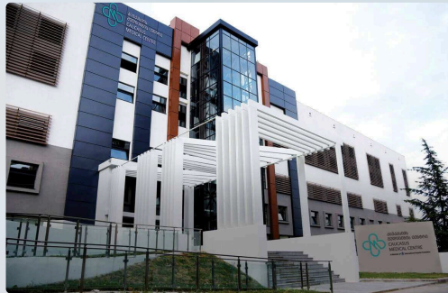
Medical Facilities Within 1 kilometer
